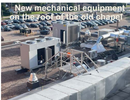
The new isolation room exhaust fan on the south wing roof
